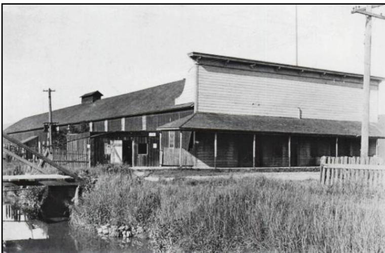
Heynemann Overall Plant at 405 First St. In Petaluma
