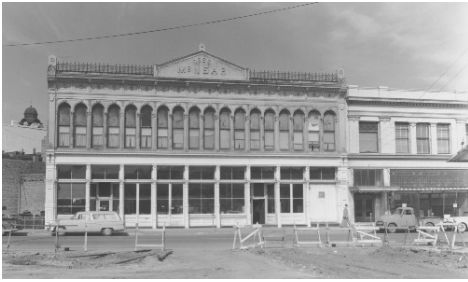
The McNear Building, constructed in 1886, displays its Victorian Italianate commercial style in 1954
