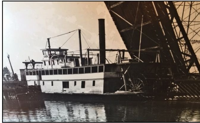
Petaluma III under D St bridge
